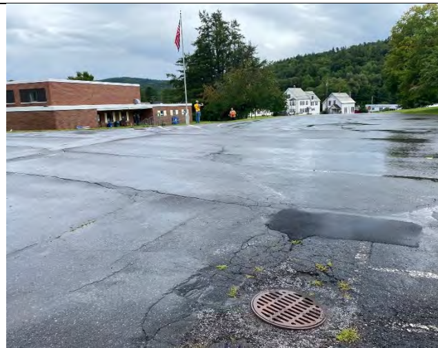
Photo 1: Catch basin tied into the system.
