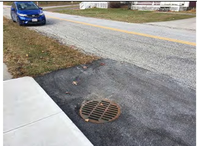
Photo 2: Road draining to catch basin
