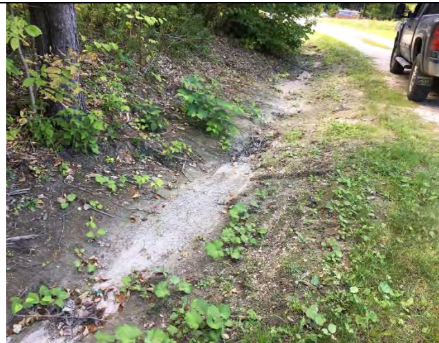
Photo 1: Sediment deposition in the swale.
