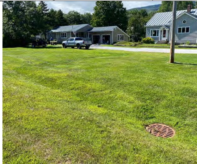
Photo 1: Drop inlet and grass swale where project will be installed.
