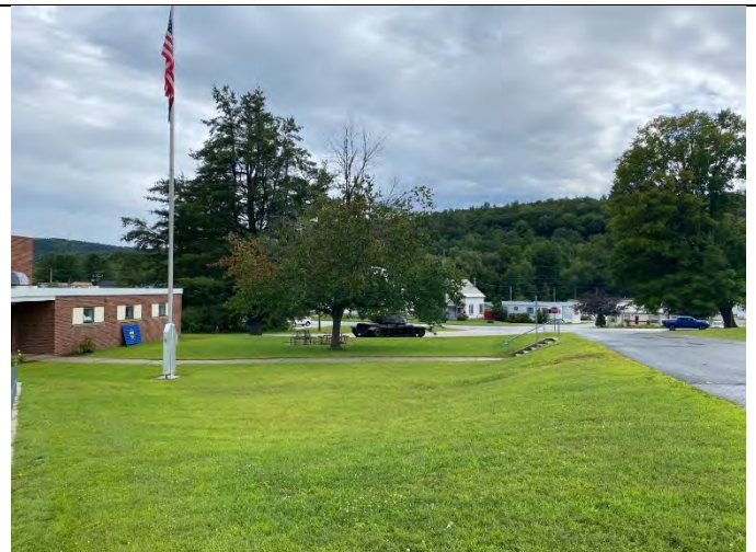
Photo 2: Green space above pipe where underground infiltration could be installed.
