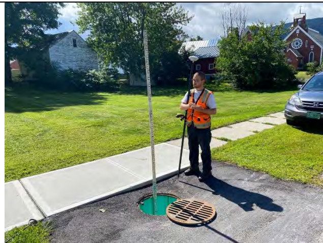
Photo 1: Catch basin next to empty lot.
