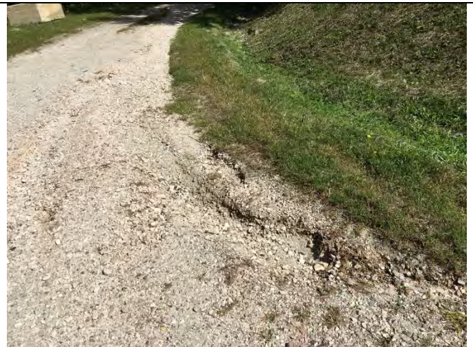
Photo 2: Eroding corner of the gravel road.
