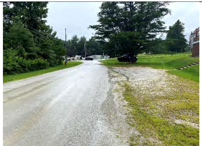
Photo 2: Erosion and sediment deposition along road in front of community center
