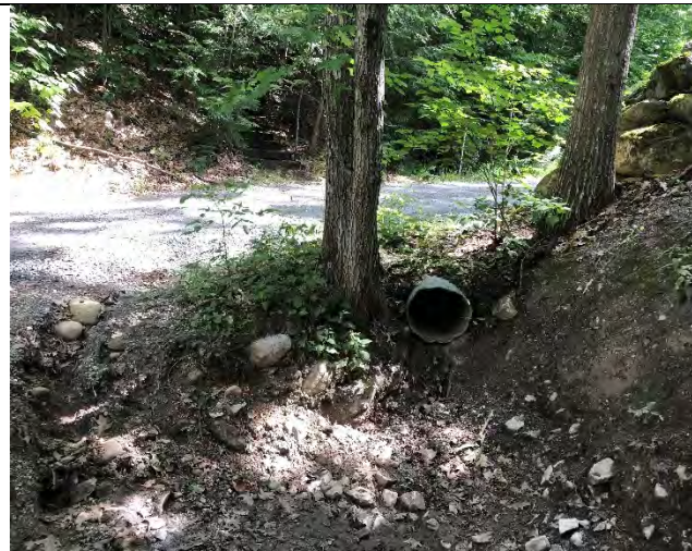
Photo 1: Outfall into eroding gully that leads to lake. Photo 2: Existing gully/flow path into lake.
