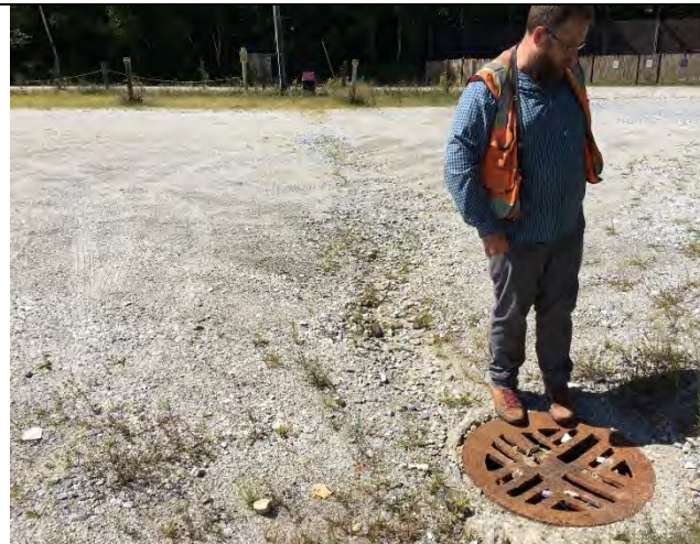
Photo 1: Catch basin in upper lot where treatment feature will be located.
