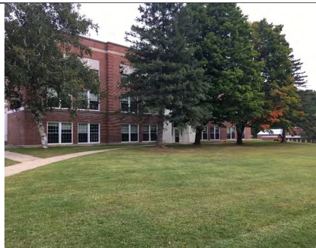
Photo 1: Open space in front of school suitable for subsurface infiltration
